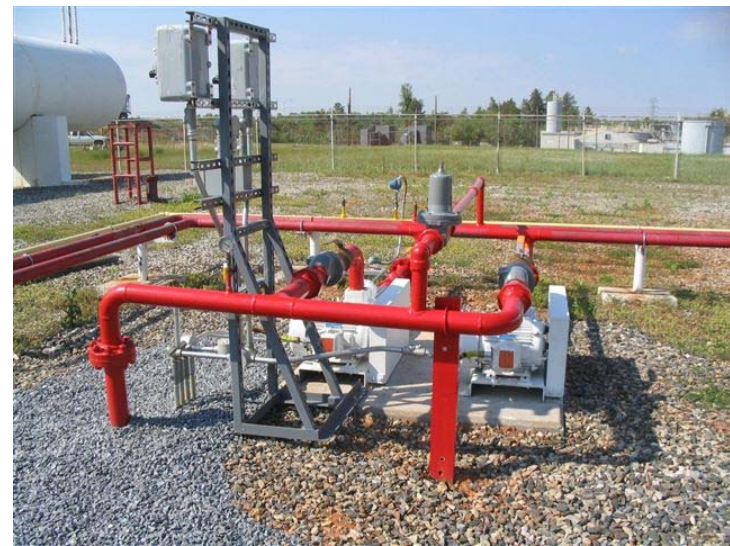
Liquid Transfer Pumps
