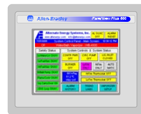
Optional EOI for Allen-Bradley PLC: 6-inch PanelView-Plus display with first-out monitor (Alarm History) and graphic TrendLine recording. Applications developed for this EOI can also run on a PC with FactoryTalk View ME Station license (for remote monitoring).
