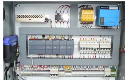
Standard Control Panel with Siemens S7-1200 PLC, Safety Relays, automatic circuit breakers, Ethernet Router, and Honeywell Flame Safeguard.
