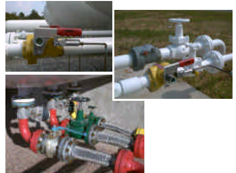
Misc. components of typical tank trim and ESVs
