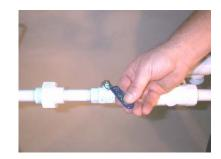
Adjust outlet regulator to desired pressure. .
