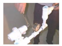
• Set outlet pressure relief valve within a range of 125% to 250% of the regulator pressure setting.
