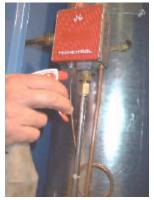
• Adjust outlet regulator to desired pressure.
